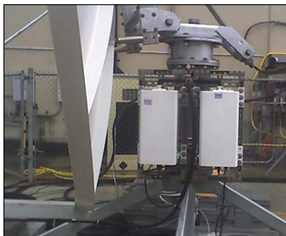
Antenna-mount 1:1 system w/ mounting frame
