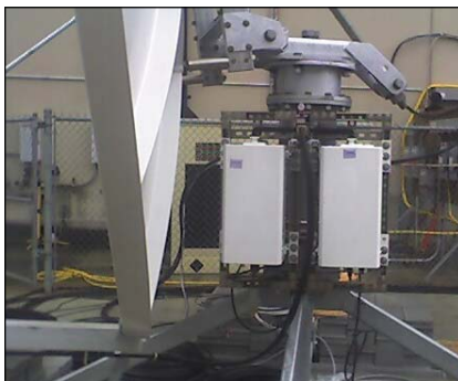
Antenna-mount 1:1 system w/ mounting frame
