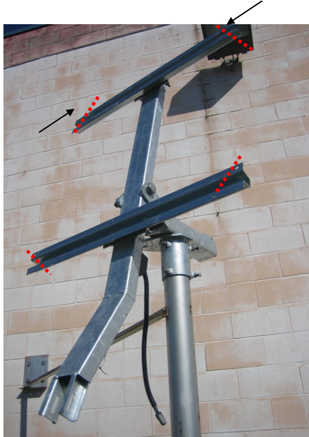
Fig. 2: Top reflector bracket installation
