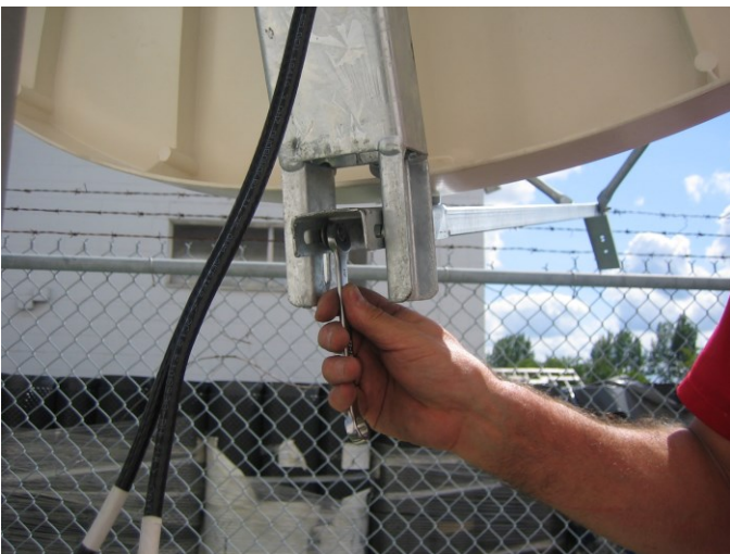
Fig. 8: Securing Feed Arm
