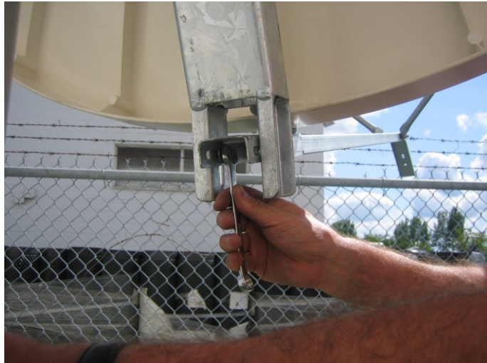
Fig. 8: Securing Feed Arm
