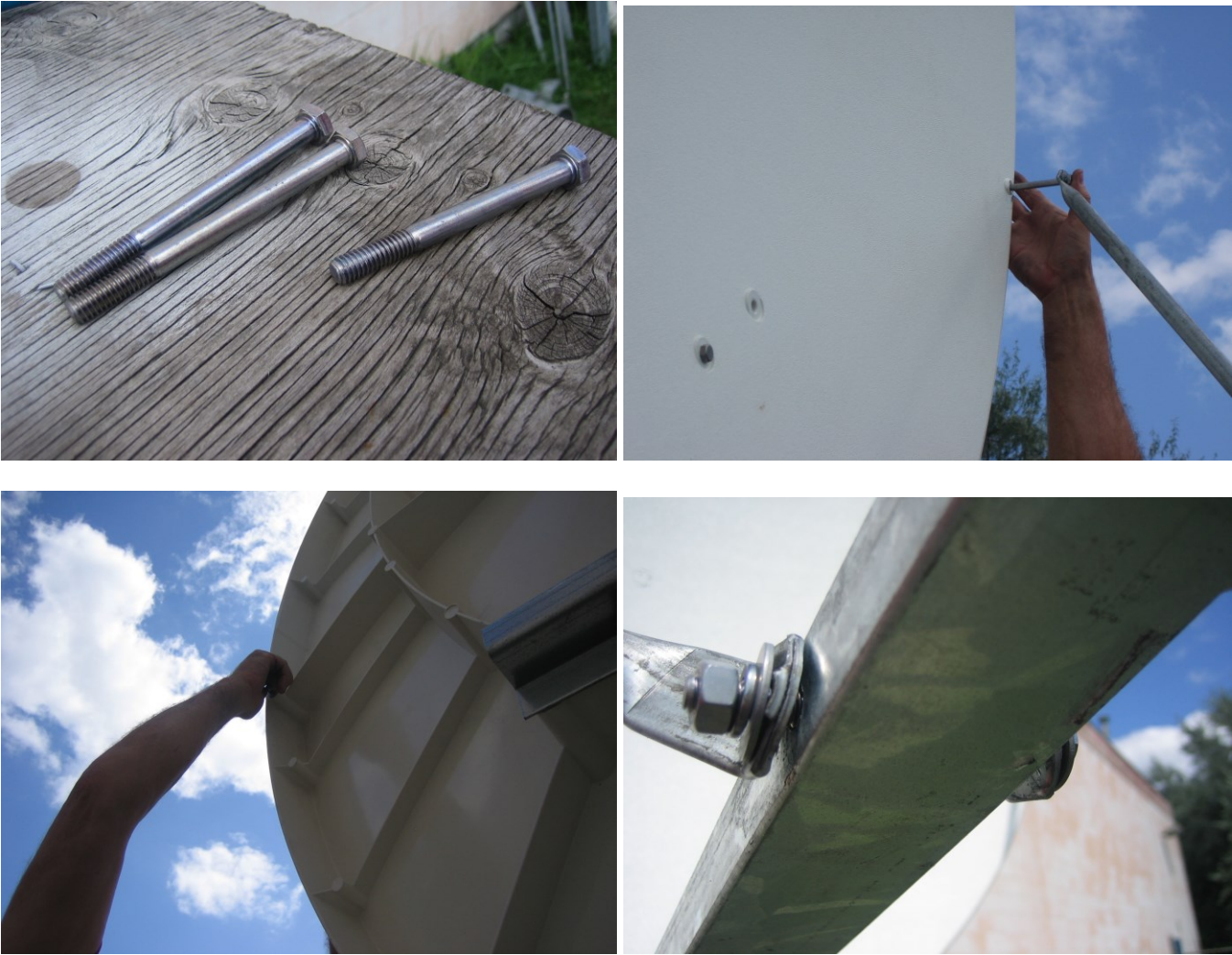
Fig. 7: Feed Boom Support bars installation
