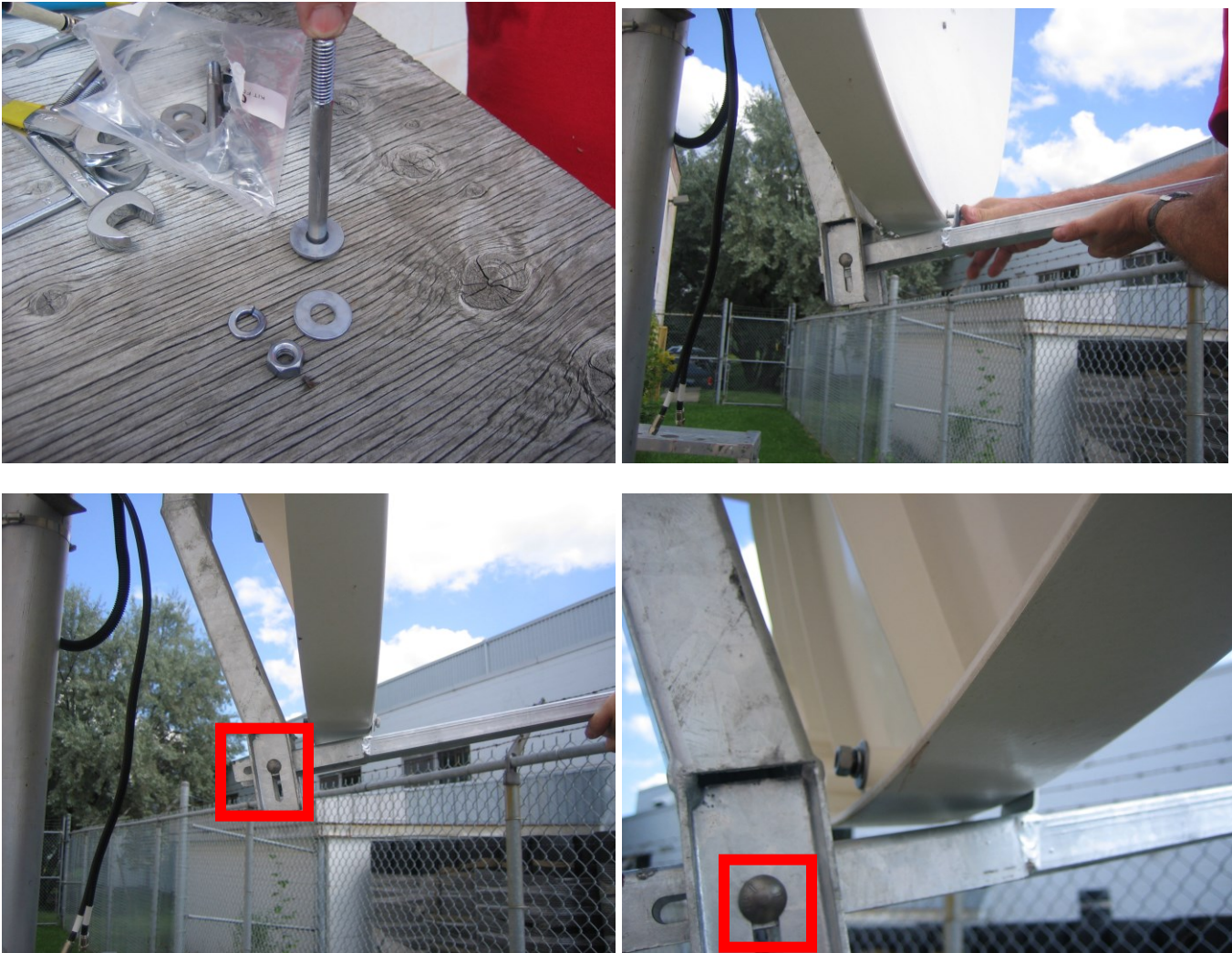
Fig. 6: Bottom reflector bolt installation
